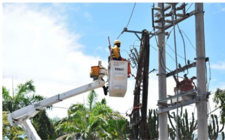
Power technician repairs a transformer.
